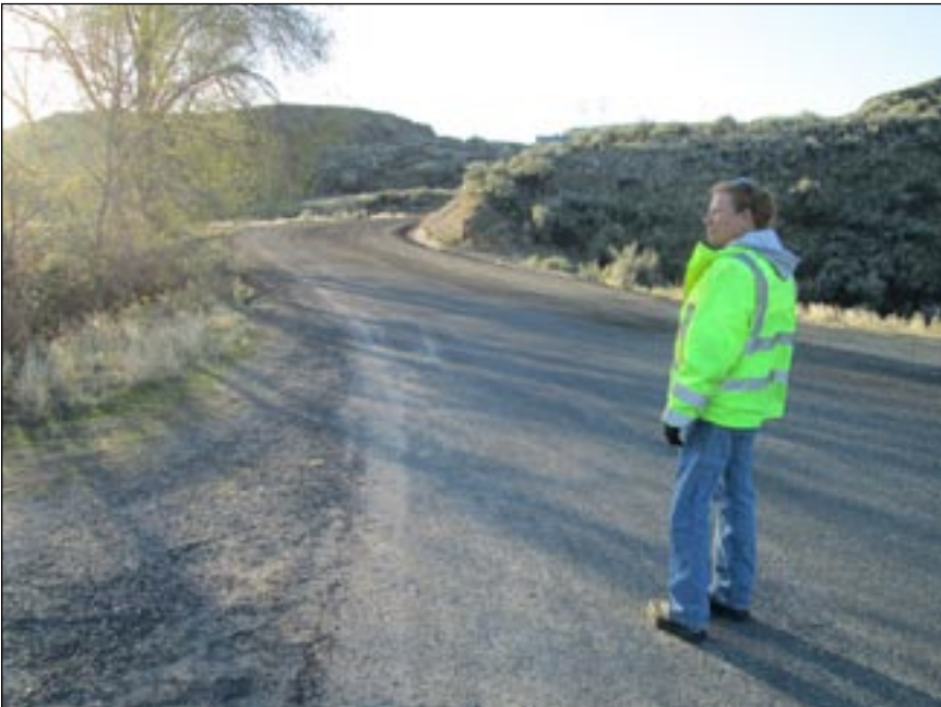
Donna Deckman, of Electric City's public works department, surveys the improvement made to Snider Road with about 50 dump truck loads of chewed up pavement from the Department of Transportation.
