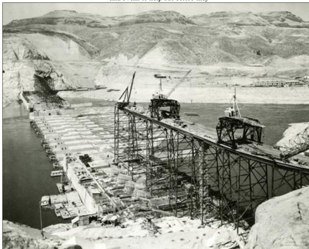
The construction trestle, with deck at El. 1180, approaches the spillway section of the dam. The Bethlehem Steel Co., under subcontract from Consolidated Builders, furnished the structural steel, and erected the trestle. August 2, 1938.
